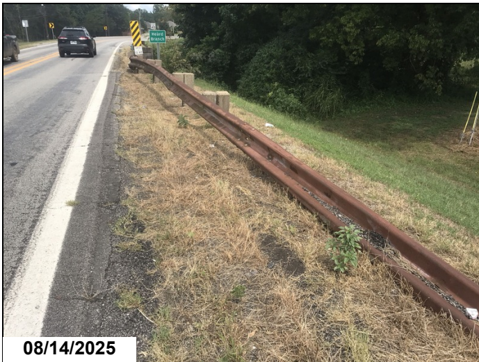
Abutment # 1, right: approach guardrail collision damage.
