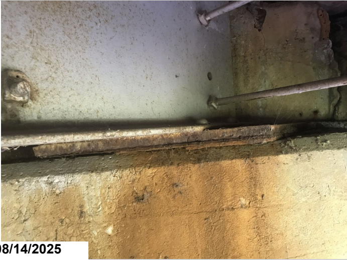
Moveable Bearings: The bearings have areas with active corrosion and layers of flaking rust.
