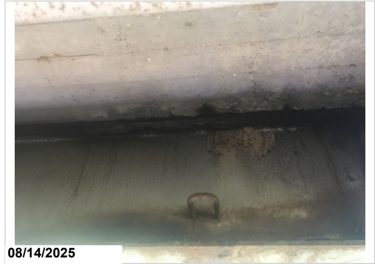
Girder # 14: The top flange of beam # 14 has an area of active corrosion with flaking rust on the exterior side near abutment # 2. Top flange appears to have approximately 1/8" section loss.
