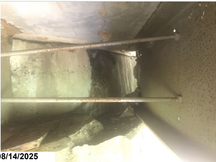
Abutment # 2, right: the backwall has a 12" x 16" spall with exposed reinforcing steel where the backwall transitions back at the wing wall juncture.
