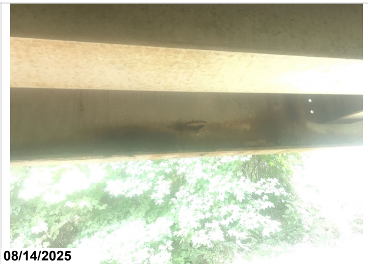
Girder # 14: girder has up to approximately 1/8" section loss to the bottom flanges adjacent to the deck drains during this inspection. The corrosion to girder #14: girder has up to approximately 1/8" section loss to the bottom flanges adjacent to the deck drains during this inspection. The corrosion to girder # 14 has section loss to bottom flange in three areas approximately 8' in length located approximately 10' from abutment # 2 that has reduced the flange thickness to 7/16" remaining section.
