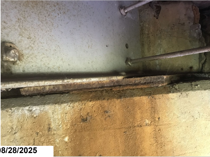
The bearings have areas with active corrosion and layers of flaking rust.
