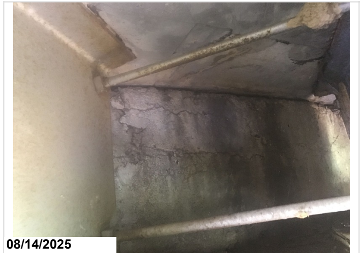
Abutment # 2: has a horizontal crack / delaminated area in the backwall behind girder # 10.
