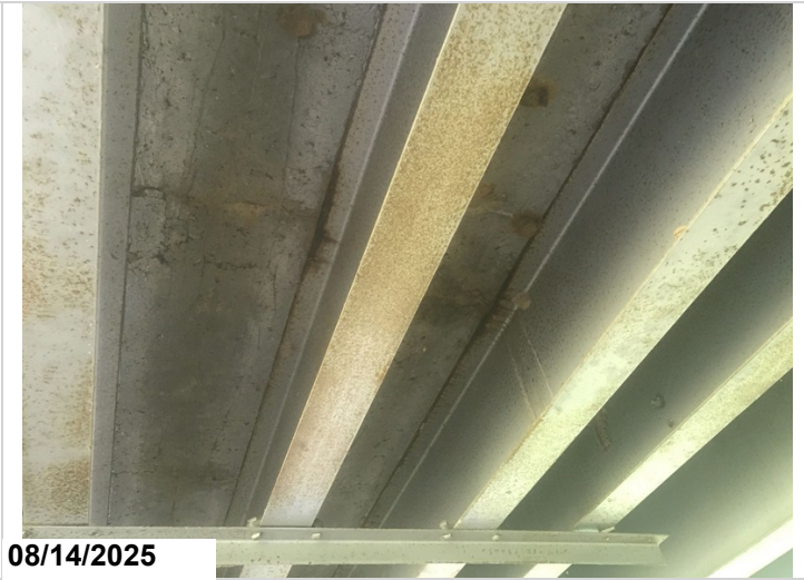
Steel Girder: top flange corrosion at full depth cracks.
