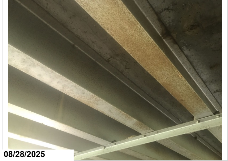
Failing paint system.
