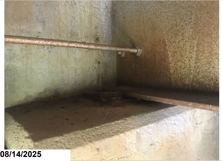
Abutment # 2, bearing # 2: active corrosion, pack rust and section loss.
