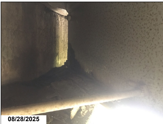
Abutment # 1, girder # 8: active corrosion, pack rust and approximately 1/8" section loss.
