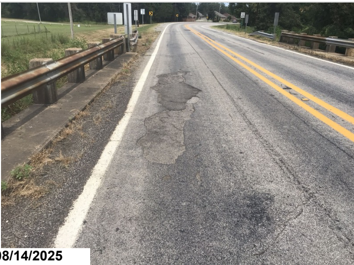
Left lane: Chip and seal wearing surface in left lane is missing in an area approximately 12' long x 2-1/2' wide.
