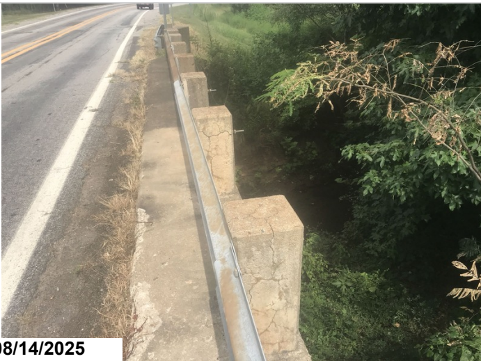
Right, posts # 3 & 4: map cracking.
