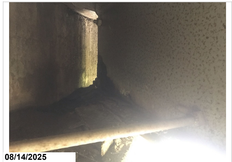
Abutment # 1, girder # 8: active corrosion, pack rust and approximately 1/8" section loss.
