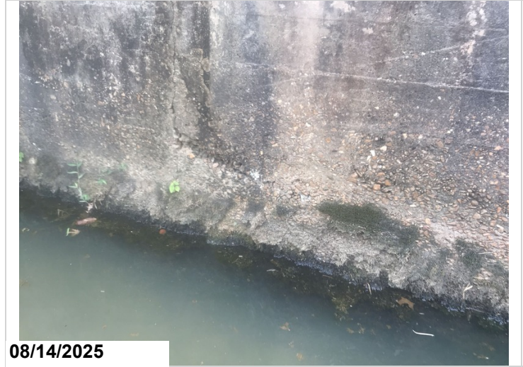
Abutment # 1, left: the left side near base of stem wall has a 16" area of shallow concrete deterioration with no exposed reinforcing steel.
