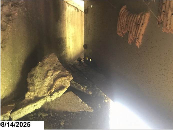
Abutment # 1, girder #2: girders have 16" of flaking rust base of web and 1/16" section loss to bottom flange in a 4" long area.
